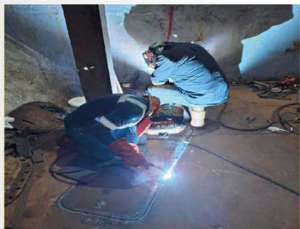
Welding Bottom Insert
