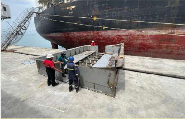
Cofferdam B Ready For Installation
