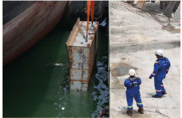
Positioning Cofferdam D
