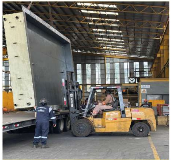
Mobilization of cofferdam A
