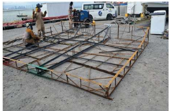
Reinforcing templates to build cofferdams
