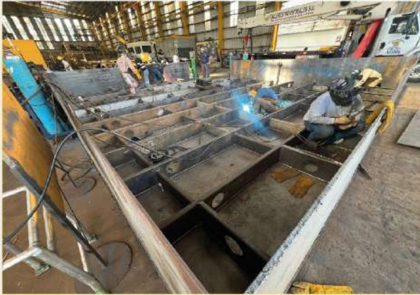
Fabrication of cofferdam A
