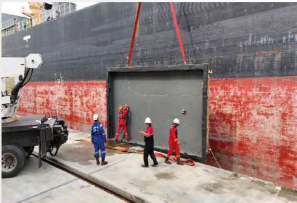
Positioning Cofferdam C
