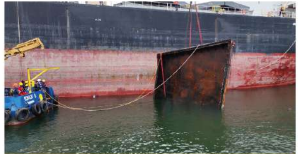
Removal of Cofferdam E
