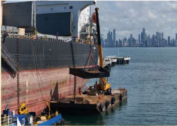
Removal of Cofferdam B
