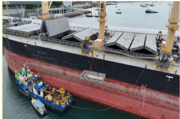
Lowering Cofferdam E
