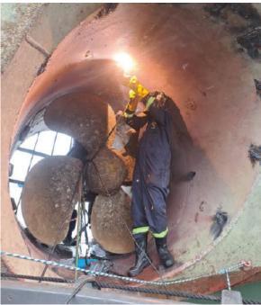
The repair was carried out afloat by trimming the vessel from the bow to get the thruster tunnel out of the water about 1mtr to allow dry repairs.
