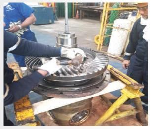
Talleres furnished skilled engineers, mechanics, and welders as well as all the necessary equipment, tools, and gears to perform the assigned jobs. We started by removing the thruster grating to allow removal from the tunnel for subsequent repairs. Propeller blades were removed from thruster to allow safe removal operation.
