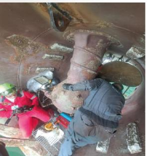
Our certified welders installed pad eyes to help our riggers lifting the thruster. Also, a beam was welded on the tunnel and used to remove the shaft. Thruster was taken to the workshop and dismantled to perform a detailed inspection, reconditioning, and replacement of needed parts.
