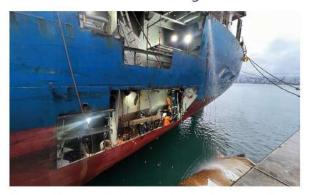
More than 40 tons of steel as well as accessories were renewed. Shell plates, frames, longitudinal frames, and brackets were renewed.
